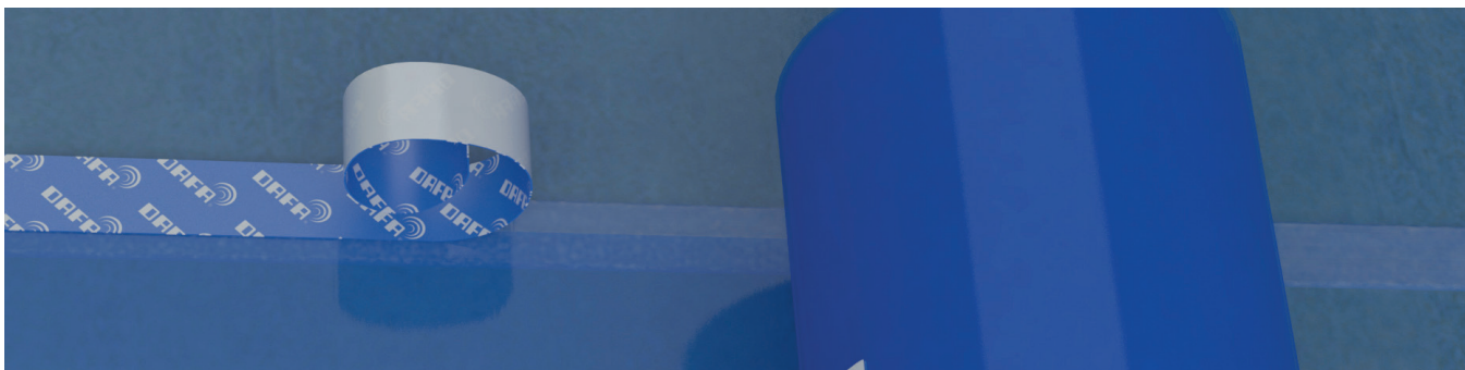
Mount the vapour barrier foil with overlaps and tape with DAFA vapour barrier tape.
