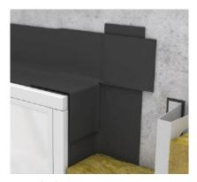
EPDM for flashing is UV resistant and is sealed around openings with EPDM adhesive.
