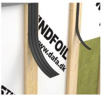
EPDM strips protect the wood behind them against the effects of weather and accomodate potential movement.
