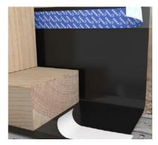
Rubber skirtings on plinths give an excellent seal and will not slip, even if the building elements move.
