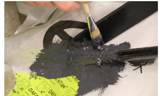
Easy seal of complex joints. Can be basted and sprayed.
