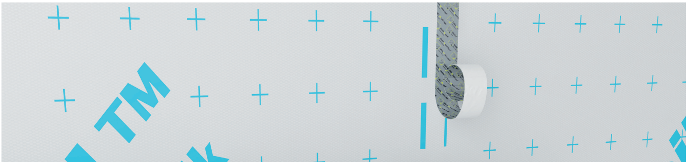
Mount the vapour barrier foil with 100 mm overlaps and tape with DAFA Hi-tack vapour barrier tape.
