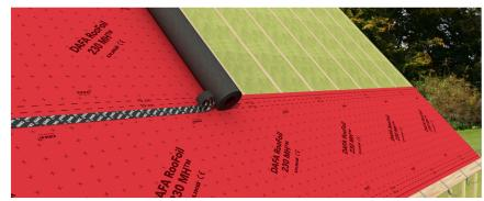
DAFA RooFoil 230 MH is installed with min. 150 mm overlay, and joints can be taped with DAFA UV tape.
